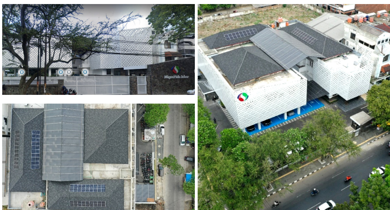
Figure A1. Headquarters of BUMD Migas Utama Jabar (previously Migas Hulu Jabar), installation of rooftop solar power plants
